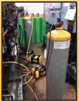
**Below:** G5Twin used daily in a reclamation facility for tank to tank transfers
