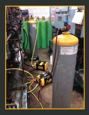
On a R-407A system retrofit of a low temperature ice cream case, the G5Twin recovered 600 lbs of R-22 in record time using the Push-Pull Method.
